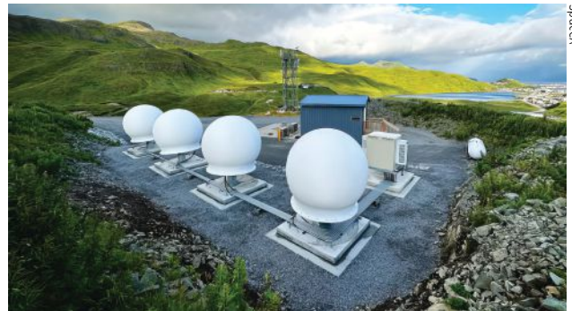
STARLINK'S GATEWAY TERMINALS are positioned worldwide, so remote areas without terrestrial infrastructure can access high-speed internet.
